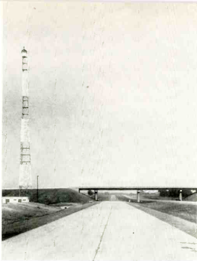
This microwave relay station serves the Indiana Toll Road, one of the most recent of the nation's super-highways to be opened to the public. Backbone of the private communications network is a General Electric Microwave system, supplemented by GE VHF mobile equipment.
